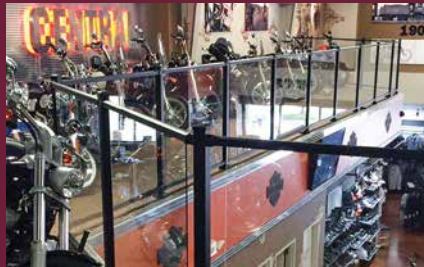
Retail Balcony Veranda Railing
