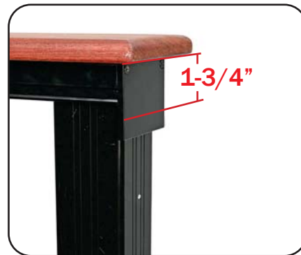
(2) Mark Reference Line Measure down 1-3/4" from the top of the extended end plate and mark a temporary line. (Keep end plate tight to post)
