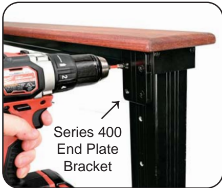
(1) Attach End Plate Bracket Attach End Plate Bracket to Rail. Attaches with 4 ea. included screws. (Grooves help to center the bracket)
