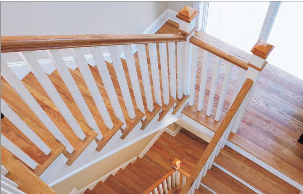
Pictured with 5360 balusters and 6310 handrail.
