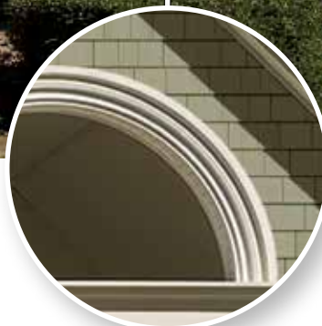
Multiple profiles used in heat formed application.
