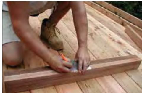
Step 2: Cut top and bottom rails (2x4s) to length and clamp together. Starting from the center of the rails, mark out 4-1/2" on-center using a tape measure or marked speed square. This will leave a 3-3/4" opening from baluster to baluster, once the balusters are installed.
