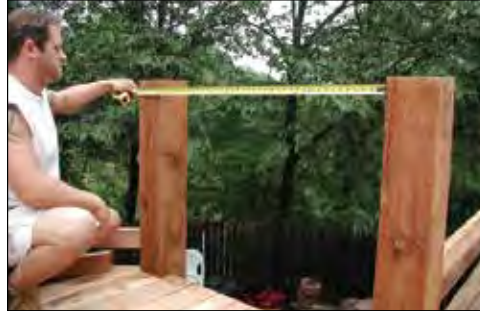
Step 1: Measure railing opening, from post to post.
