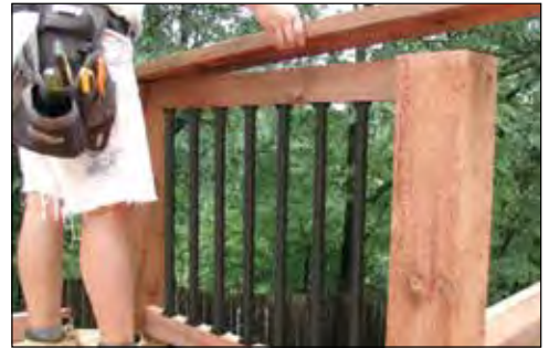
Step 5: Place top rail (2x4) over balusters. Install cap rails for a finished look.
