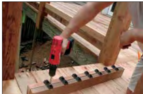
Step 3: Screw on Deckorators Estate baluster connectors (sold separately) on each mark.
