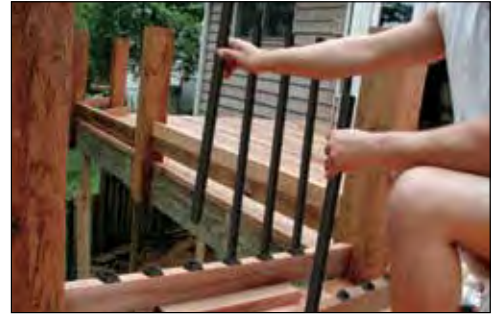
Step 4: Place the bottom rail (2x4) on 1-1/2" blocks (2x4 scrap material works best) and attach to the post. For easy rail-to-post connection, we recommend using Deckorators railing connectors (sold separately). Put clear adhesive on each connector to properly secure balusters and prevent spinning. Insert balusters over baluster connectors.
