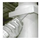
STEP 16: Apply construction adhesive to the cap and base.
