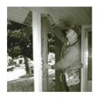
STEP 2: Using a jack and post, jack up the beam only enough to remove the existing post, no more than 1/4".
