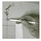
STEP 4: Hang a plumb bob from the top centerline to determine the bottom centerline.
