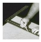
STEP 6: Using a square, draw a centerline perpendicular to the outside edge of the platform.
