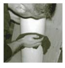
STEP 21: Remove dust by wiping the column, cap, and base with soap and water.
