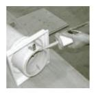
STEP 14: Apply construction adhesive to the top and bottom of the column.
