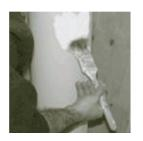
STEP 22: Paint the column with a highquality oil-base or acryliclatex paint.
