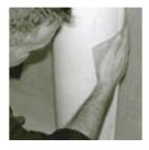
STEP 20: Prepare the column for painting by sanding lightly with 120-grit or finer wet/dry sandpaper.
