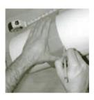
STEP 9: Using a piece of cardboard as a guide, draw a line all the way around the column.
