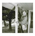
STEP 1: Measure the total distance from the bottom of the beam to the platform.
