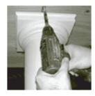
STEP 15: Put the assembly in place and plumb. Make sure that the load is centered over the column shaft and evenly distributed. Secure L-brackets to the platform and beam.
