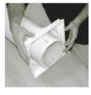
STEP 12: Slide cap over the top of the column to rest on the neck ring, then slide the base onto the column.
