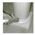
STEP 19: Apply caulk to gaps between the cap and base and the column shaft.
