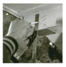
STEP 3: Determine the top centerline and mark it on the beam.
