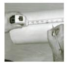
STEP 8: Measure from the top of the column to the proper length and make a series of marks around the column shaft.
